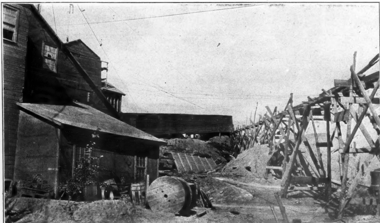
Trough Down Which Dust Collected from the Crushing and Screening Operations is Washed
